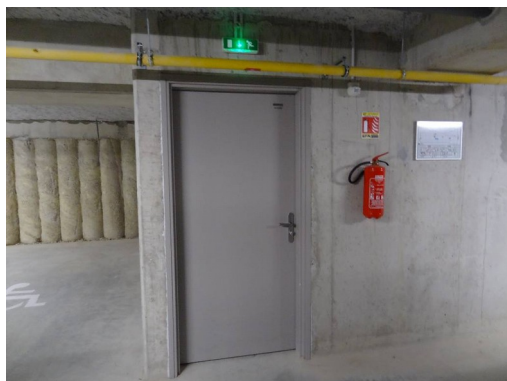
Absence couple foyers lumineux
