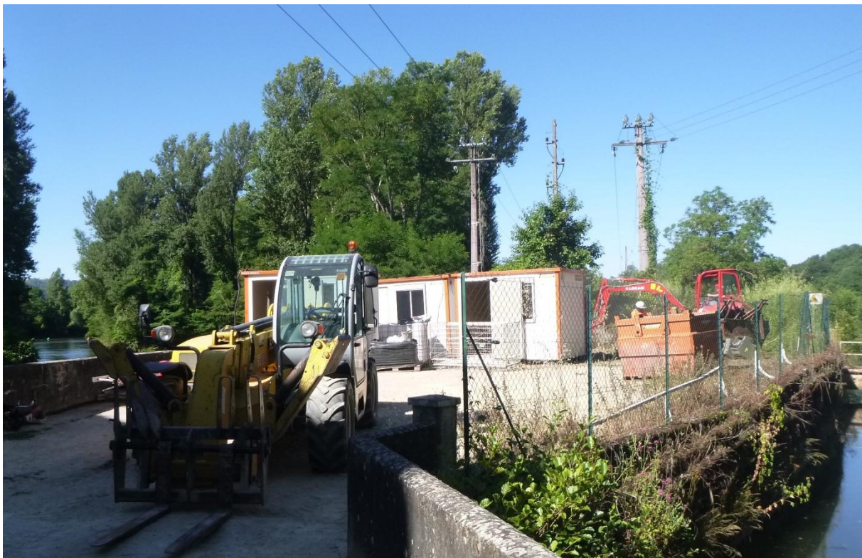
Figure 18 – Installations de chantier 2016
