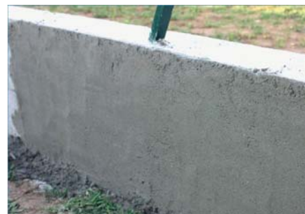
Mur parpaing - habillage ciment
