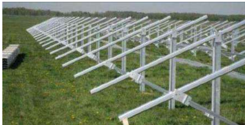
Figure 10 : Structures de support sans modules
