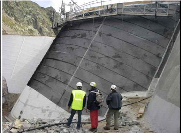
**Figure 13 : Mise en place de la géogrille**
