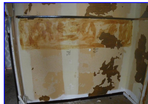
Joints de Placoplatre
