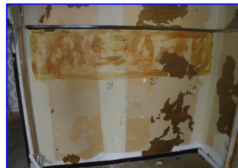
Joints de Placoplatre
