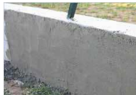
Mur parpaing - habillage ciment
