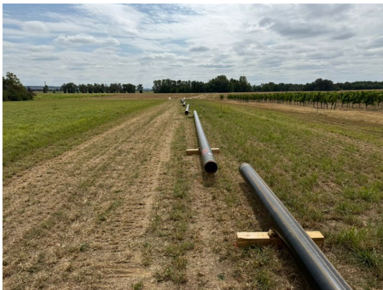
Figure 71 Bardage des tubes
