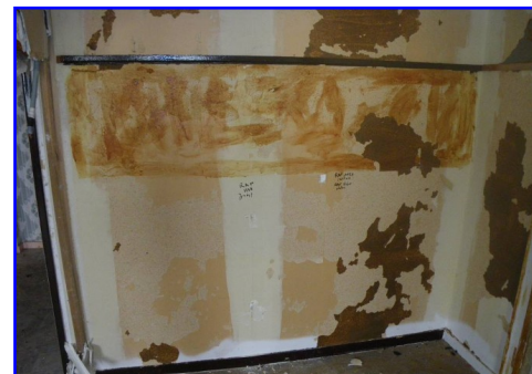
Joints de Placoplatre
