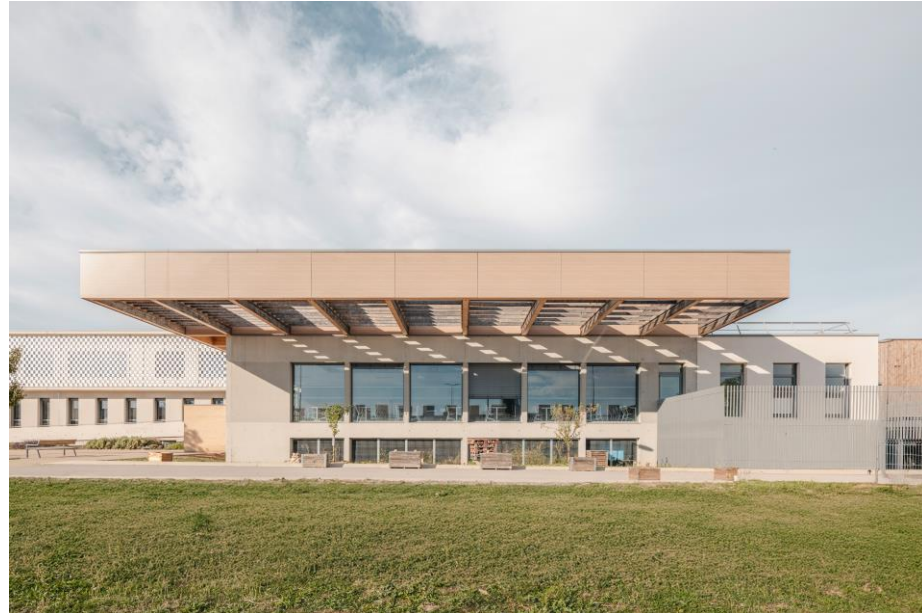
Façade SUD Restauration
