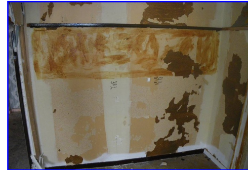
Joints de Placoplatre
