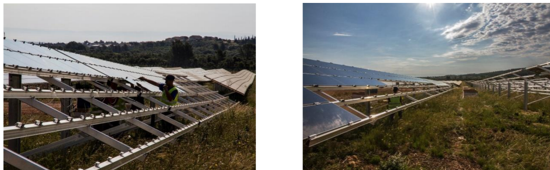
Figure 12. Montage des structures supports (source : NEOEN)
